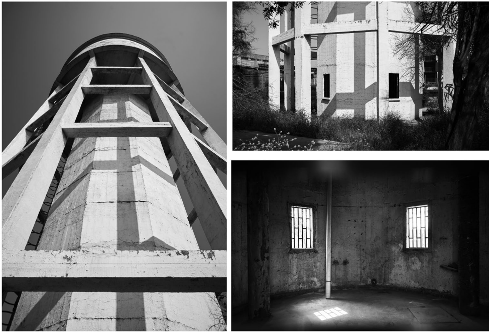
Figure 3. Quinta Bella's water tower. Left: Exterior of water tower. Top right: Ground level of water tower. Bottom right: Interior of water tower. Photos by the authors, 2022.
