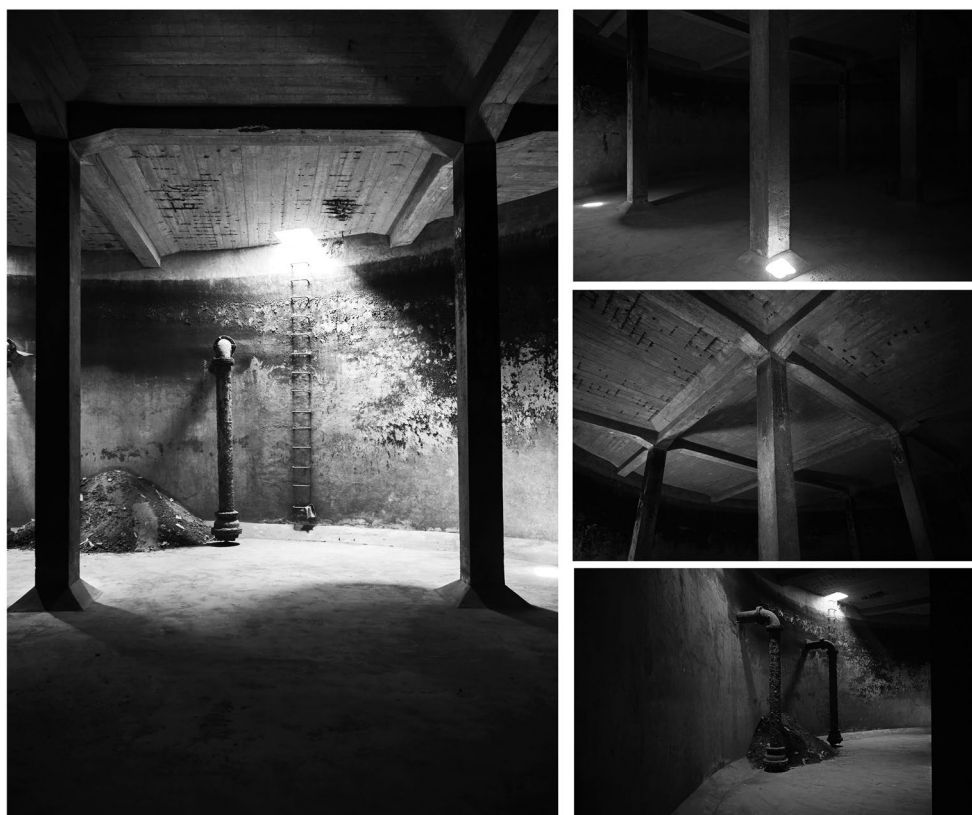
Figure 6. Interior of the water reservoir. Top right photo by the authors, 2022.
